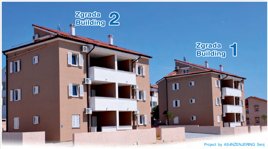
DVIJE POTPUNO ISTE ZGRADE, SVAKA SA 11 APARTMANA. TWO COMPLETELY SIMILAR BUILDINGS, 11 APARTMENTS IN EACH.
